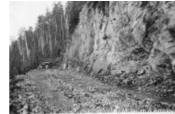
Building the R/R grade Hill 60 (2020_06_08_004)
