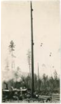
Spar tree showing rigging yarder and donkey engines (2020_06_08_001)
