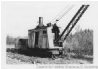
Vintage self propelled steam crane at Paldi (2020_06_08_03_005)
