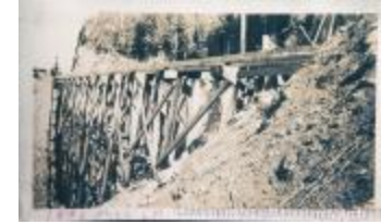
R/R bridge on Hill 60 (2020_06_08_02_001)
