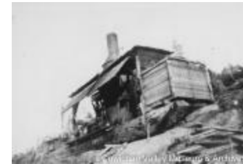
[A donkey engine on a lumber yard] (2020_06_08_05_003)
