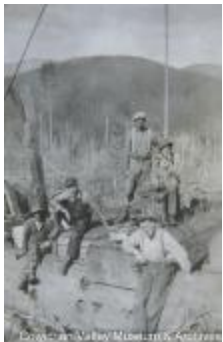
[Five unidentified loggers pose on logging machinery] (2020_06_08_05_004)
