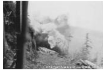
Blasting for R/R on Hill 60 (2020_06_08_003)
