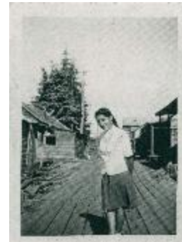
[Photo of Deepo K. Sardar on the boardwalk, Paldi, B.C.] (2023_09_01_01_12_012)
