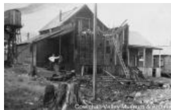
[Unidentified man standing next to damaged building] (2020_06_07_242)
