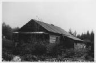
[A wooden house surrounded by bushes and trees in the background] (2020_06_10_001)
