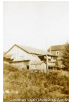
[Two wooden buildings] (2020_06_10_023)
