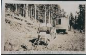
[Photo of gas shovel transporting fuel] (2023_09_01_02_02_015)
