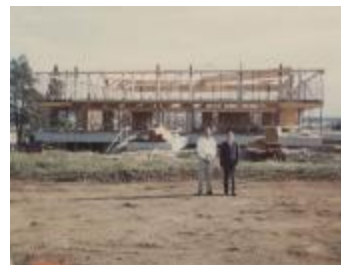
[Photograph at Ross Street gurdwara building site] (2022_15_01_025)
