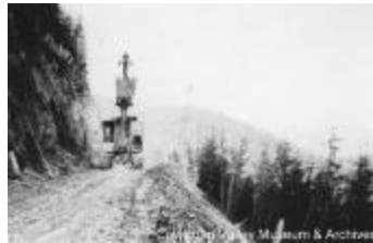
[Perry Ross and his North West gas shovel building more railroad] (2020_06_08_03_002)
