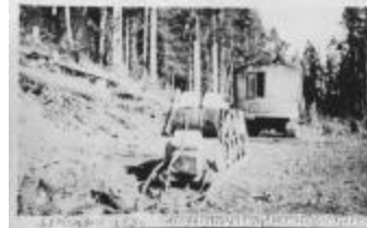
[Perry Ross and his North West gas shovel building more railroad] (2020_06_08_03_003)
