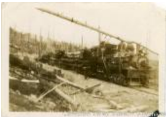
Train load of logs going to mill (2020_06_08_06_010)
