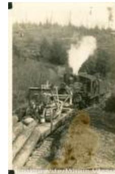
Moving heavy equipment and logs at Kapoor operation (2020_06_08_06_001)
