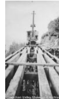
Extending the rail line on Hill 60 (2020_06_08_03_004)
