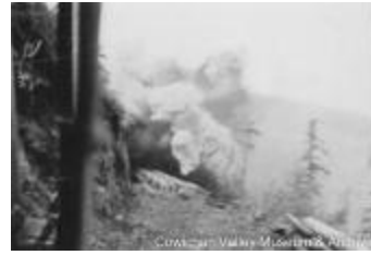
Blasting for R/R on Hill 60 (2020_06_08_003)
