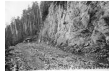
Building the R/R grade Hill 60 (2020_06_08_004)
