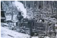
[A Mayo Lumber Co locomotive] (2020_06_08_06_003)
