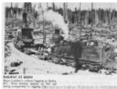
Mayo Lumber Co. locomotive transporting a donkey engine (2020_06_08_06_005)
