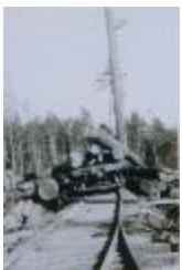
[Photo of a flat car being loaded with logs] (2023_09_01_02_02_019)
