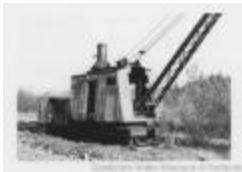
Vintage self propelled steam crane at Paldi (2020_06_08_03_005)
