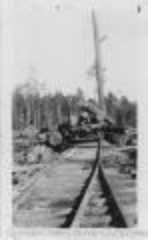
Logs being loaded on flat car (2020_06_08_04_006)
