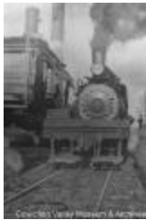
Taking on water (2020_06_08_07_003)
