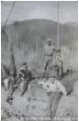
[Five unidentified loggers pose on logging machinery] (2020_06_08_05_004)
