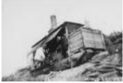
[A donkey engine on a lumber yard] (2020_06_08_05_003)
