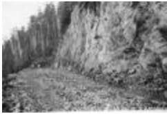
Building the R/R grade Hill 60 (2020_06_08_004)
