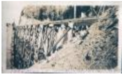
R/R bridge on Hill 60 (2020_06_08_02_001)
