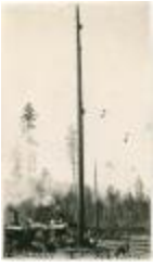
Spar tree showing rigging yarder and donkey engines (2020_06_08_001)
